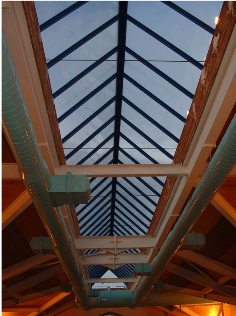
FIGURE 7 Roof of Bedale Leisure Complex swimming pool showing 316 tie bars.
