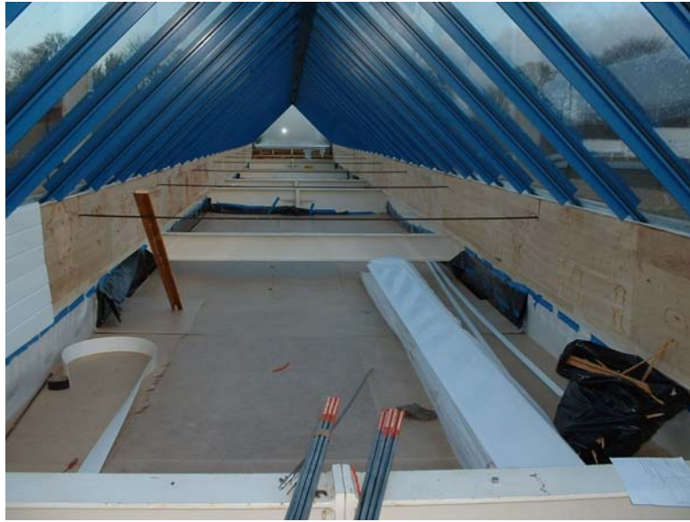
FIGURE 8 Zeron 100 tie bars awaiting installation in swimming pool roof.
