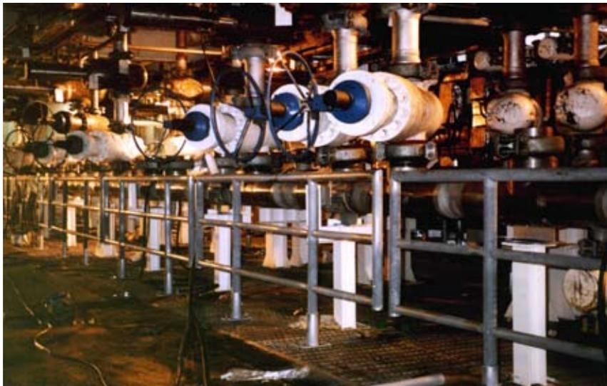
**FIGURE 6 Header and pipework in Zeron 100 on the Phillips Embla Platform**
