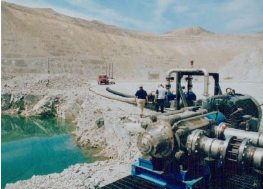
Figure 7 A Zeron 100 pump in a copper mine in the USA
