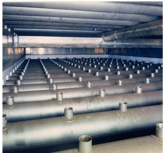
**Figure 3: N08367 Alloy Spray Piping**
