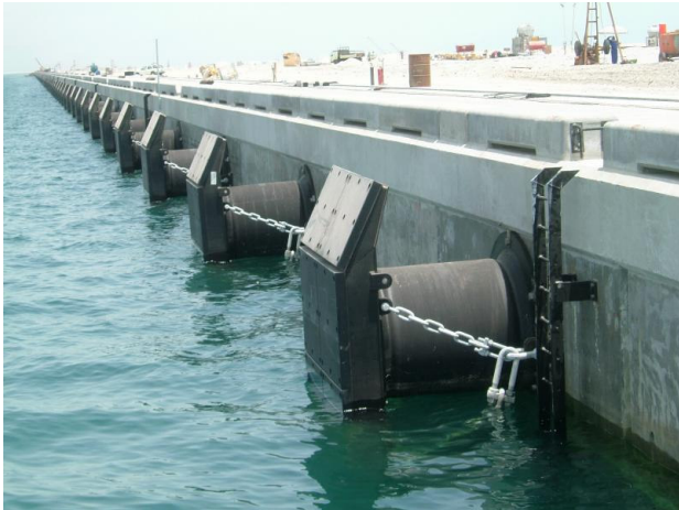
Figure 2 Z100 bolting on fenders on a dock in Bahrain
